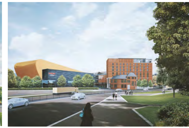
APPROACH FROM A63 WEST
